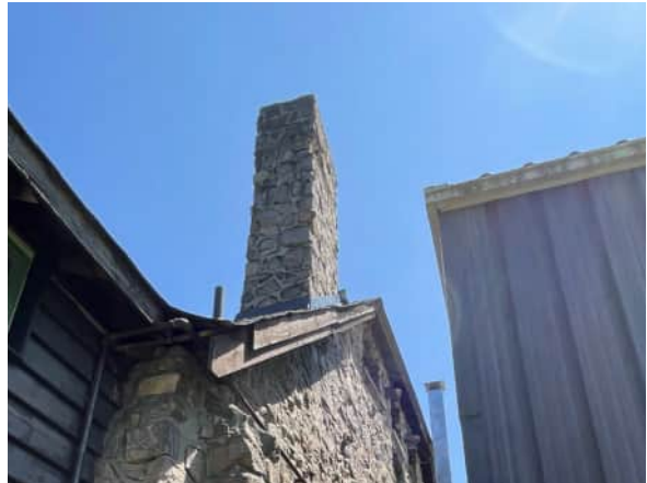
The fieldstone chimney stack on the west elevation (ERA, 2023).
