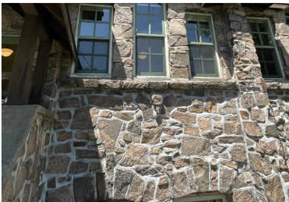
Primarily naturally-shaped fieldstone masonry with thick mortar, cut stone lintels and rusticated granite window sills (ERA, 2023).
