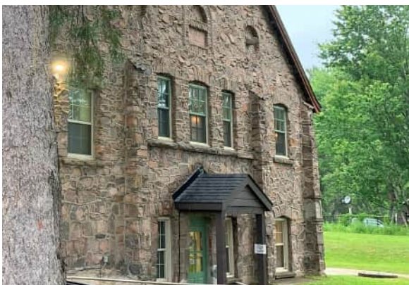
Half height fieldstone piers on the east elevation (ERA, 2023).
