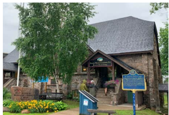
Full height fieldstone piers and stone entrance walls on the principal (south) elevation (ERA, 2023).
