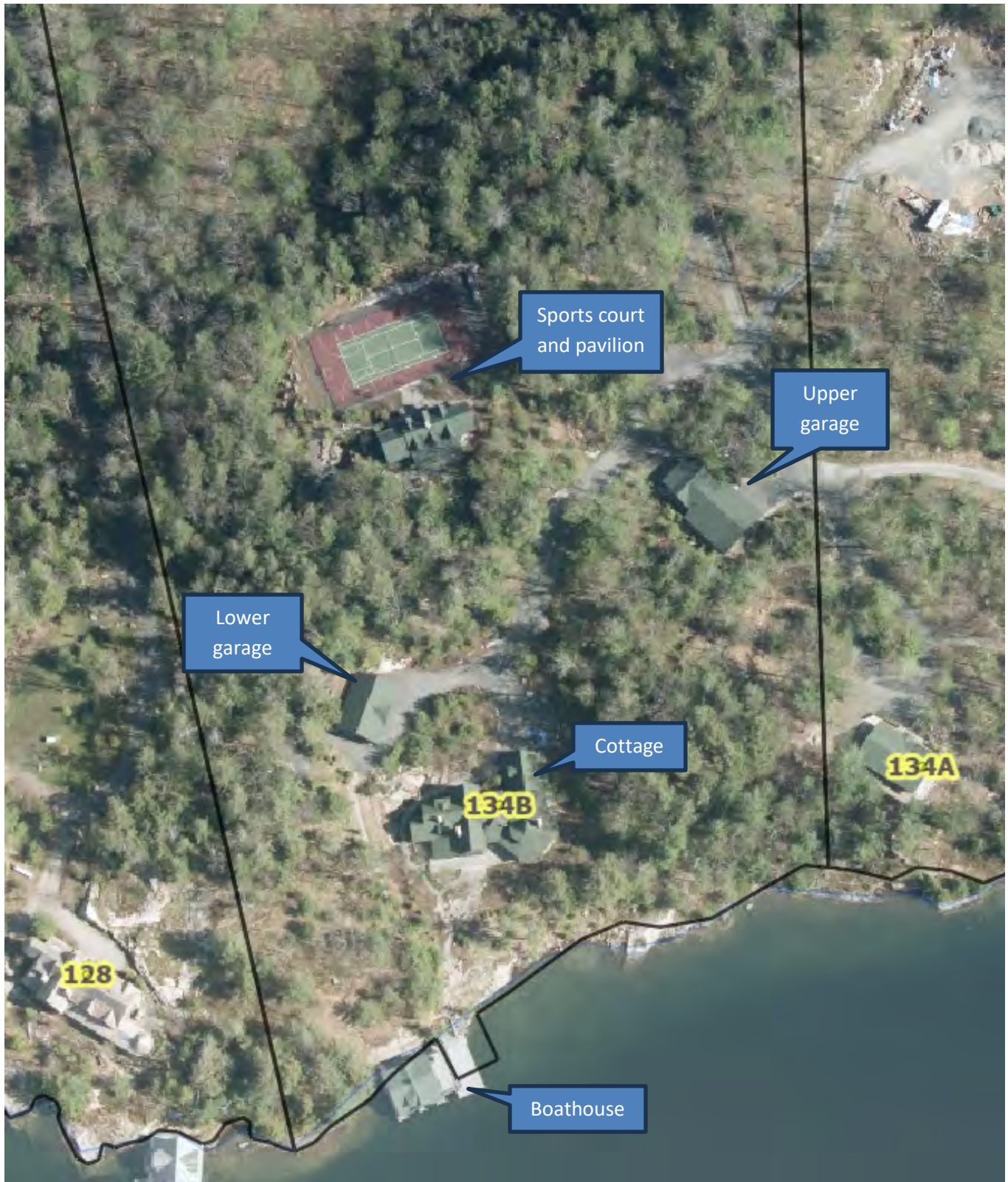
Figure 2: Air Photo of Subject Lands (south portion developed area)
